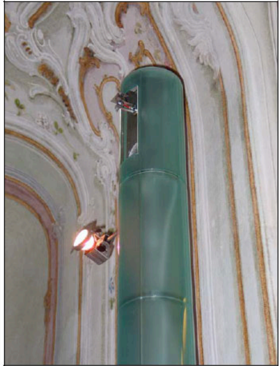
Schloss Schonbrunn, Vienna: Service pillar with integrated water sprinkler head (Photo Ingval Maxwell)
